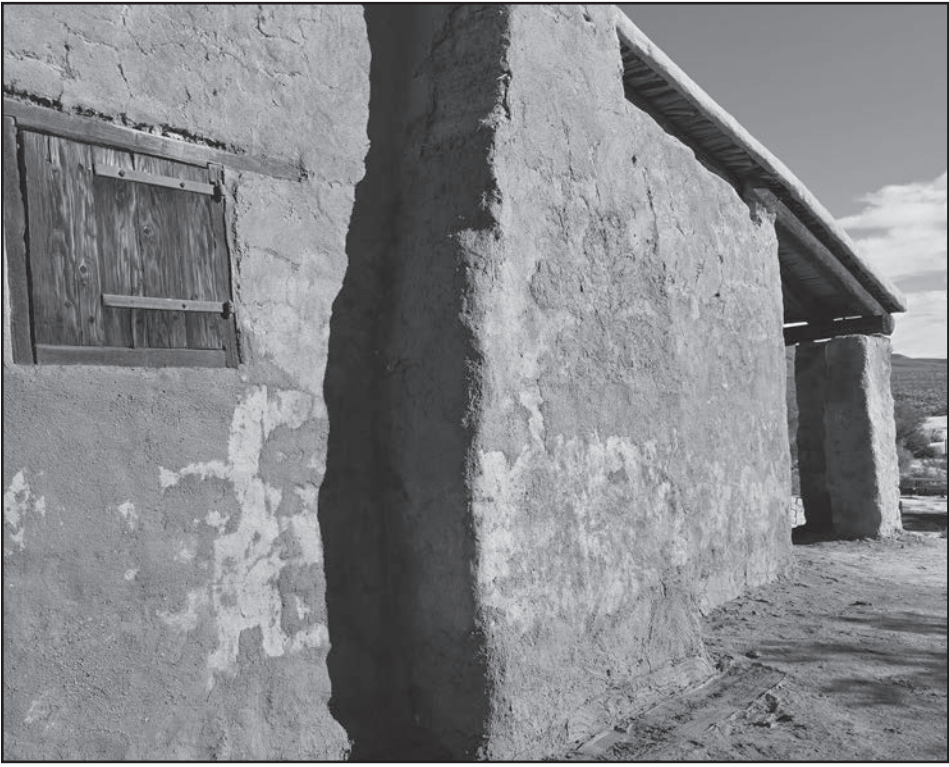
Volunteers scraped away the damaged blocks and mud, replaced with new blocks, then applied a protective layer of mud to the exterior.
